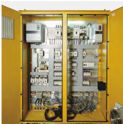
Figure 4: Example of a switching installation for the automation of machines and systems, each with a share of the power section and control section.
